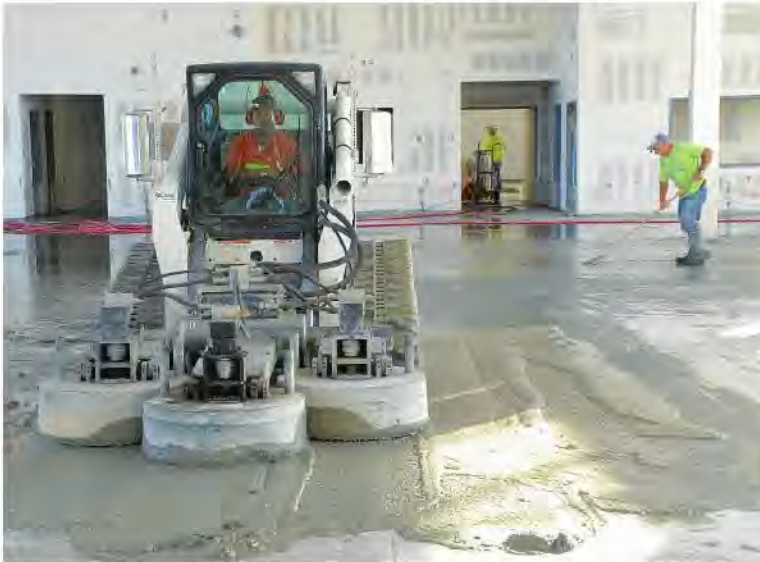
The equipment used to produce a ground, honed, and polished concrete floor should not only create a uniformly finished floor from wall edge to edge, but also promote high productivity, wet-cutting, and reduced environmental impact.
