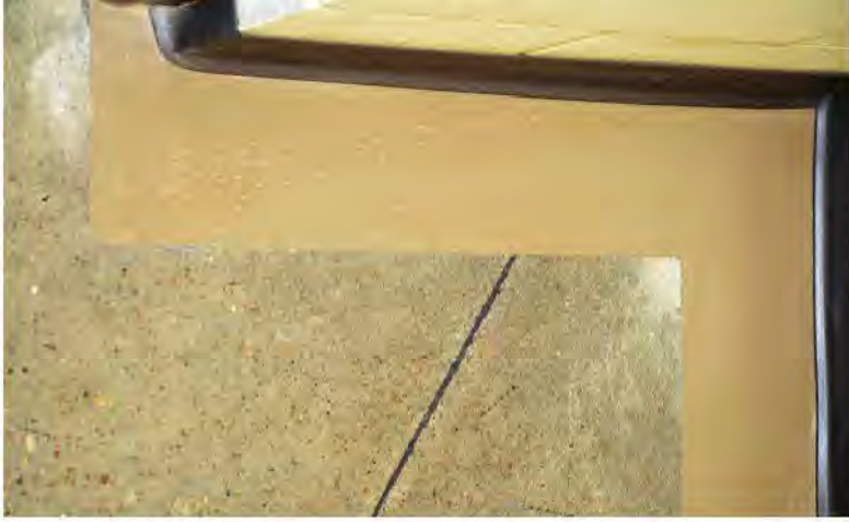
There is a need to specify a processed floor to the wall edge, as opposed to adding change orders that do not meet client expectations.
